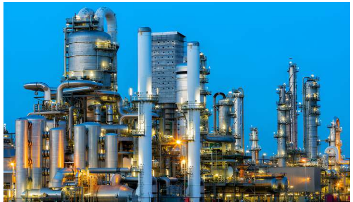
PETRO CHEMICALS, REFINERIES, OIL & GAS INDUSTRIES
